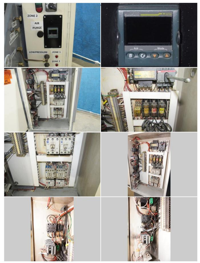
**Description:** Used, Mokon Model MK4815-BG 30 kW (15 kW per zone) Dual (two) Zone Portable Hot Oil Process Heater Temperature Control Unit with Cooling Water Circuit For Sale, Features include: Eurotherm 3216 controllers, Water Cooling Circuit, Built-in pump pressure relief valve, Unit on casters for easy movement, Mokon Dependability, , Eurotherm 3216 Controls, Second Hand, DCM-4770
