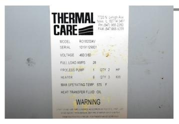
**Description:** Used, Thermal Care Model Oiltherm RO182004V 18 kW Single Zone Portable Hot Oil Process Heater Temperature Control Unit with Cooling Water Circuit For Sale, Features include: Auxiliary Water Cooling Circuit, Oiltherm RO series Digital controls, Low Profile Portable unit, Same day shipping available, ,, ThermalCare Digital Controls, Second Hand, DCM-4663
